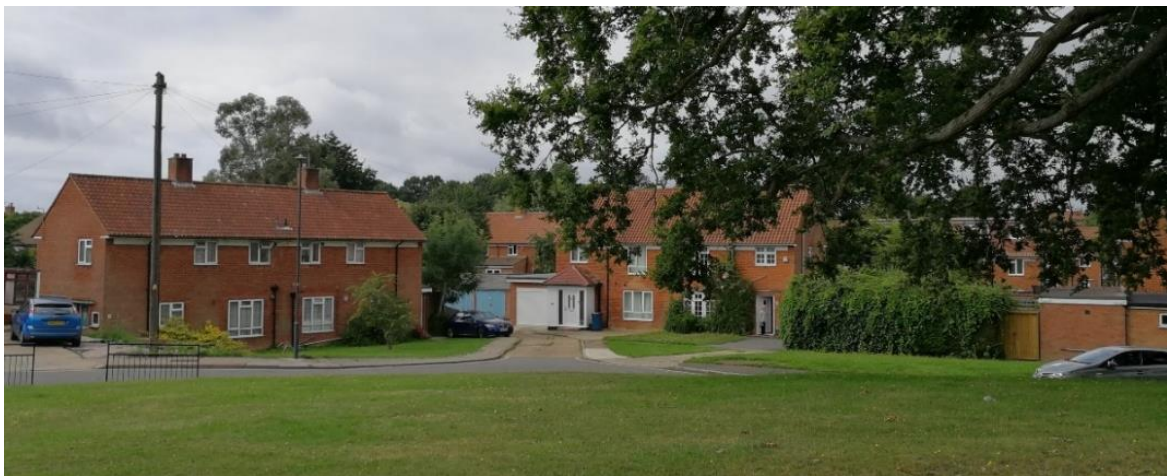
View of the site from the raised landscaped area to the north.
